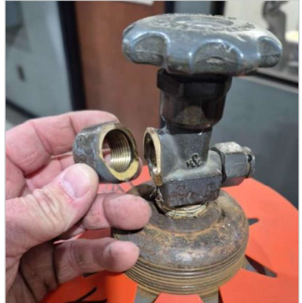
Severed valve inlet
